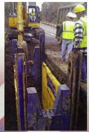
Vertical sheeting and trench support system replaces conventional application of wood or steel sheeting
